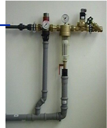
raw water inlet unit
