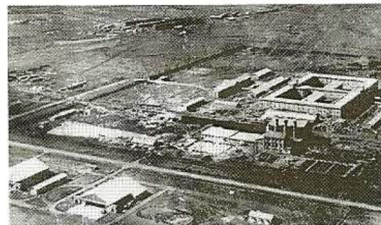
Unit 731 headquarters at Pingfan, Near Harbin in Manchuria
