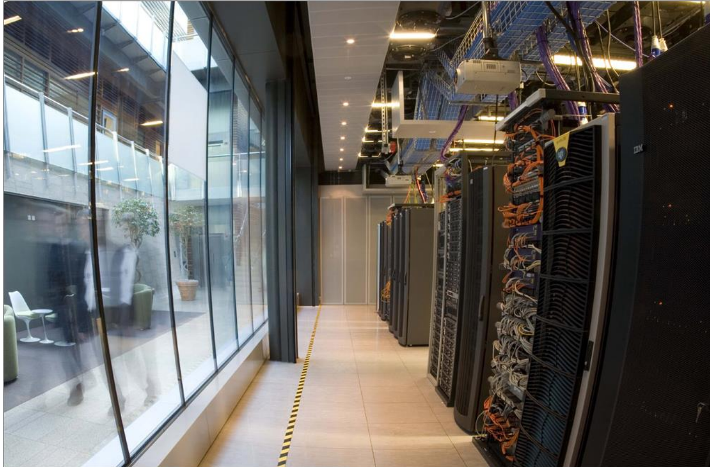
The Data Centre. The Institute's computer systems can store up to 4 petabytes of data [Credit: Genome Research Limited]
